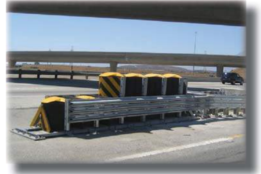
Permanent Compressor® installation at California Interstate 15N/60W interchange
