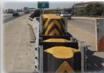
Attached to Thrie Beam Barrier
