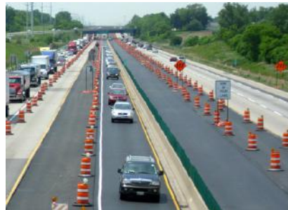
Delineate traffic lanes during resurfacing work
